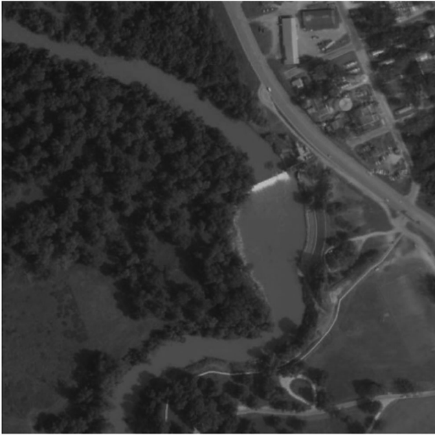
Figure 7. Widening below a run-of-river dam on the Guadalupe River at Gonzales. The channel upstream of the dam (top of photo) is 20 to 27 m wide, whereas the widened area downstream is up to 95 m wide
