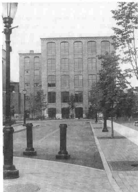
Figure 4: Refurbished street, Oil City.
